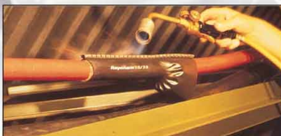
Heat shrinkable wraparound sleeve for cable sheath repair
