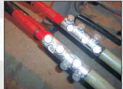
Mechanical connectors installed in straight through joint
