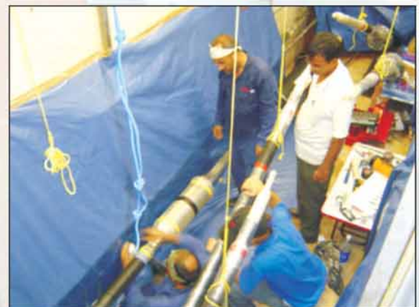
Installation of EHV cable joints
