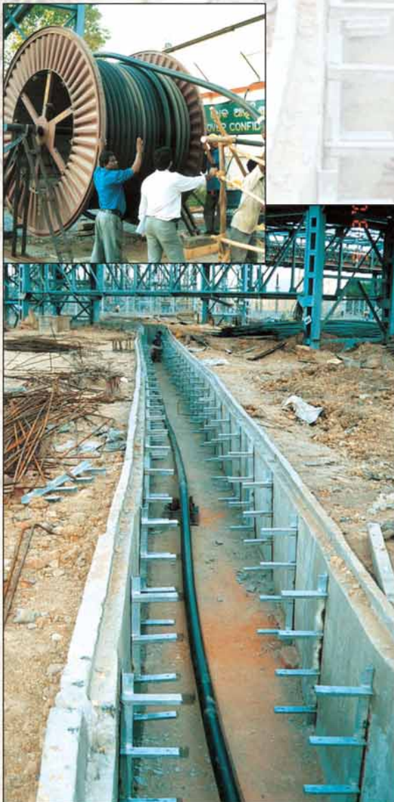
EHV 132kV cable installation work
