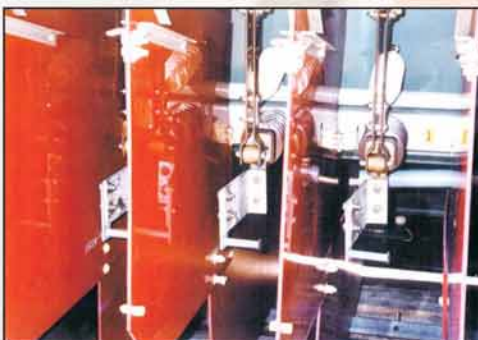
Raychem's Red Rigid Barrier Board (RRBB) used for phase segregation, to provide higher insulation and protection from flash overs.
